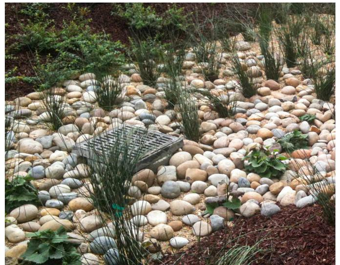
▲ **Green Infrastructure:** Rain garden and landscaping that work to reduce flooding and pollution caused by stormwater.
