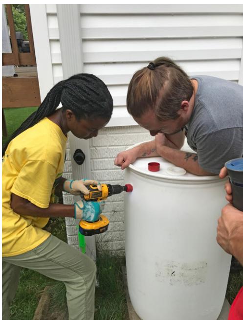
Rainbarrel preparation and installation. Photos courtesy of Howard EcoWorks.
